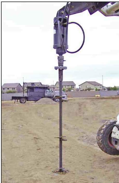
Typical MB Brace Badger Installation
