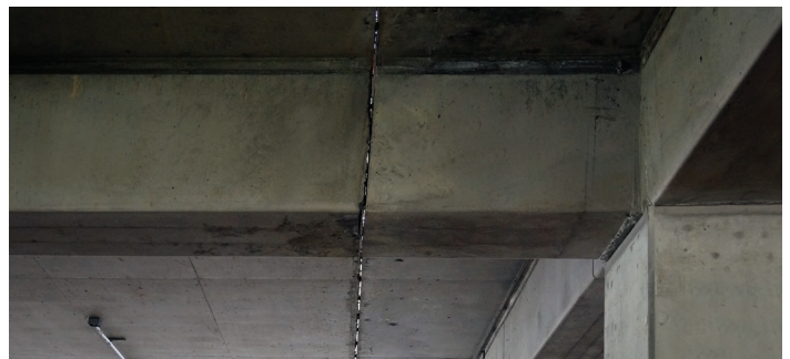
Using Burke DSD's in Beams in conjunction with slab-to-slab Burke Lockable Dowels
