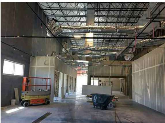
The build-out of the new corporate offices
