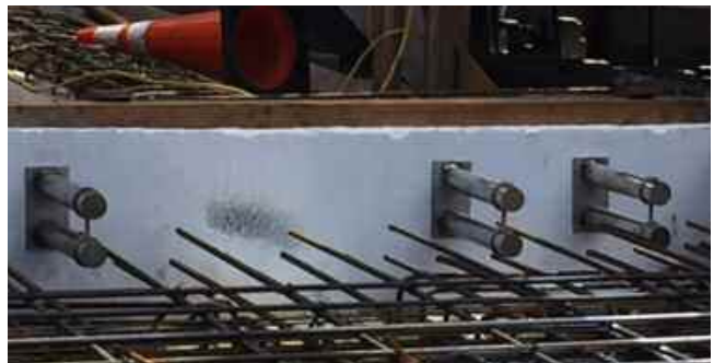
Two-part system including end plate with nail holes provides easy and accurate installation
