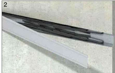
Once the formwork is removed, the steel cover will be exposed. Remove the steel cover to expose the pre-bent reinforcing steel.
