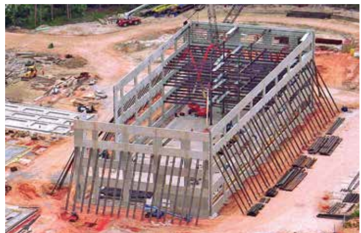
Tilt-up construction using the MB Brace Badger Helical Anchor System
