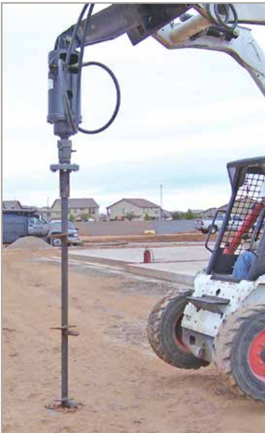
Typical MB Brace Badger Installation
